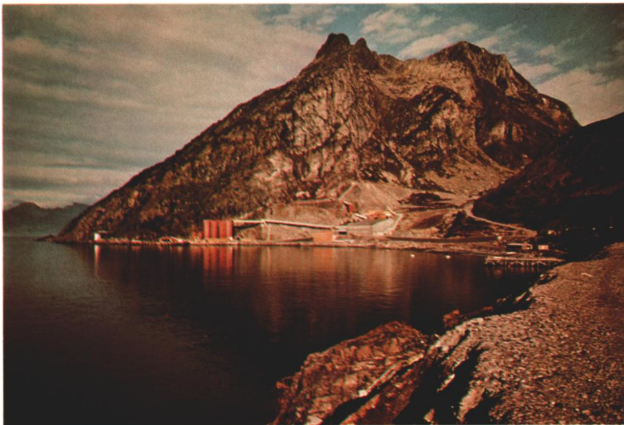
FIG. 5. Norsk Nefelin's operation of Stjernøy, northern Norway. Mine entrance is near the center of photo at an altitude of 100 m. Mine operations continue, inside Nabberen Mountain, to an elevation of 350 m. Administration building and refining plant in center foreground, quay and concentrate silos at left.
